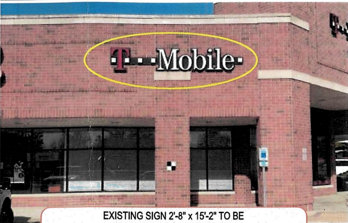
EXISTING SIGN 2'-8" x 15'-2" TO BE REMOVED & DISCARDED; WALL TO BE PATCH AS REQUIRED
